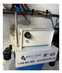
Pull the square head straight up. Be careful not to hit/break quartz tube inside the housing
