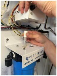
Carefully remove current lamp by gently wiggling the head unit side to side while simultaneously pulling up
